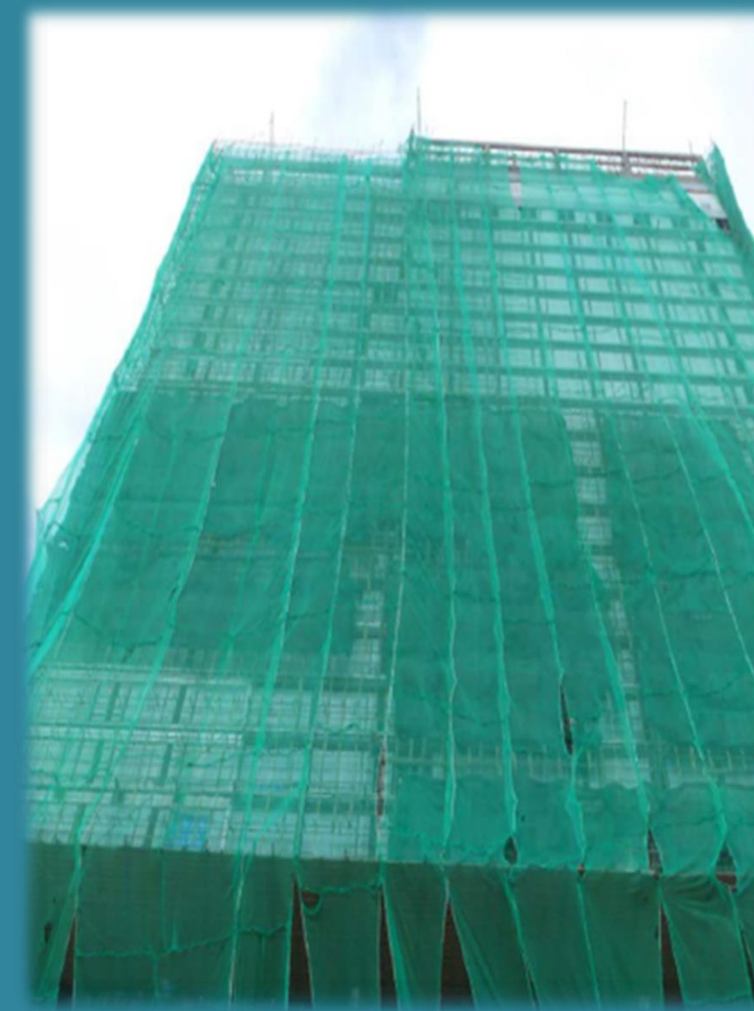
Safety Netting at Building Envelop
