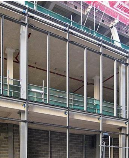
Installation of Sub-frame(1/2020)
