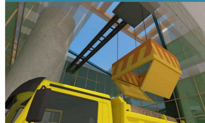
Mechanical Muck Hoist System
